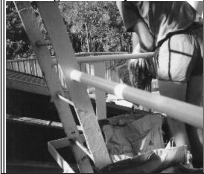
Fig 4 – Adding to a Truck Mixer
